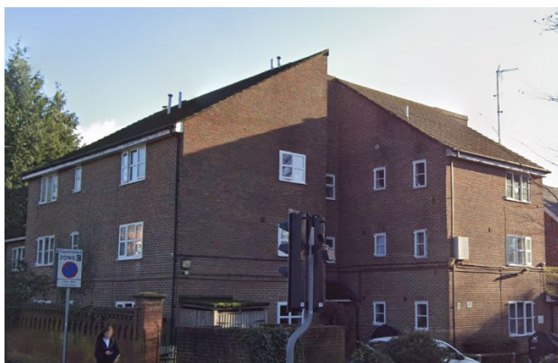
Photo 1 – Front / Flank Elevation
