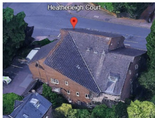
Photo 2 – Rear / Flank Elevation
