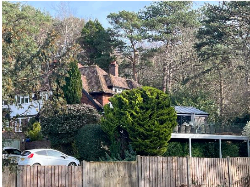
Property to rear which has had extensions - Branscombe, Heather Way
