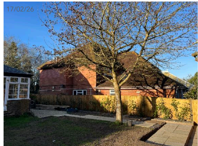
Side Elevation of Bainbridge Court (note two storey extension)
