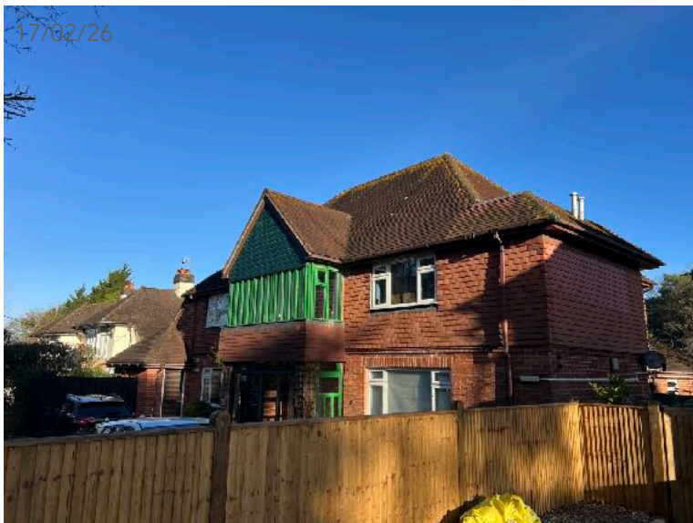
Front Elevation of Bainbridge Court (note two storey extension)
