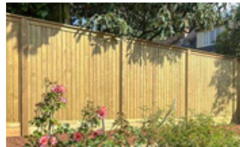
1.8m timber separation fence with concrete posts
