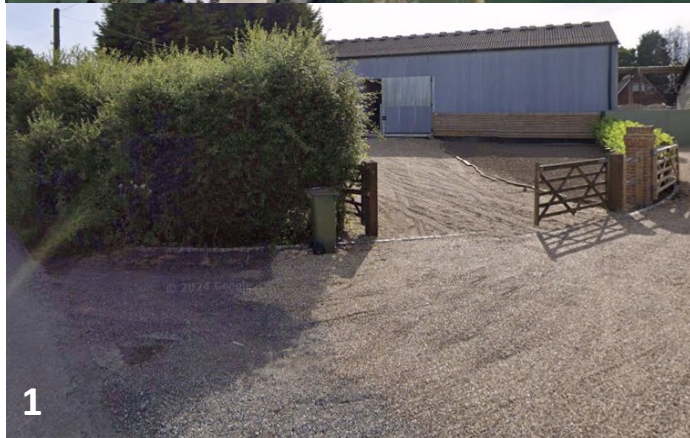
Sincox Lane at entrance to site
