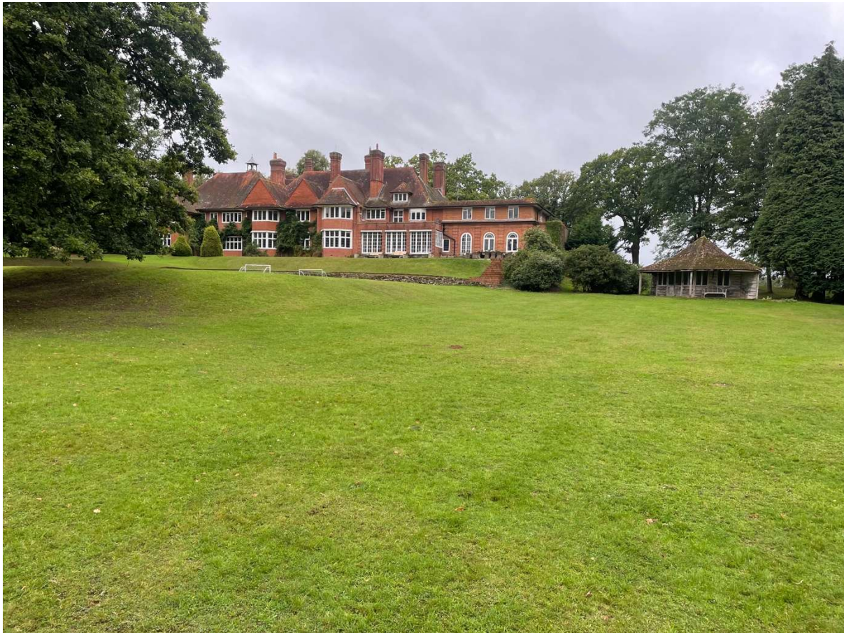
The image above depicts the original parkland gardens, which remain unbroken and intact alongside House 2b. In the top right corner of the picture, the existing summer house, rhododendron bushes, and fir tree create a natural boundary with the gardens of House 2a
