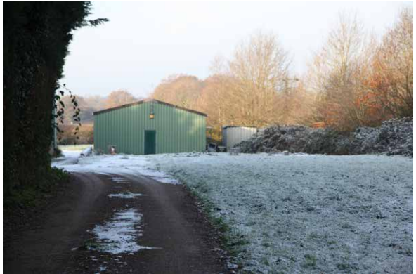
View into Site showing large sheds in eastern parts of site
