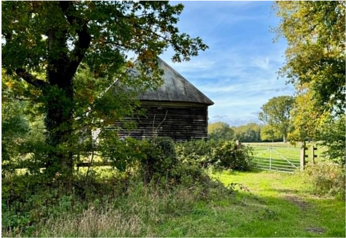
Fig 3: The east facing side elevation of Town Barn as seen from Dragons Green Road, which benefits from existing vehicular access into the proposed site. From this aspect, the proposals will broadly preserve its setting.
