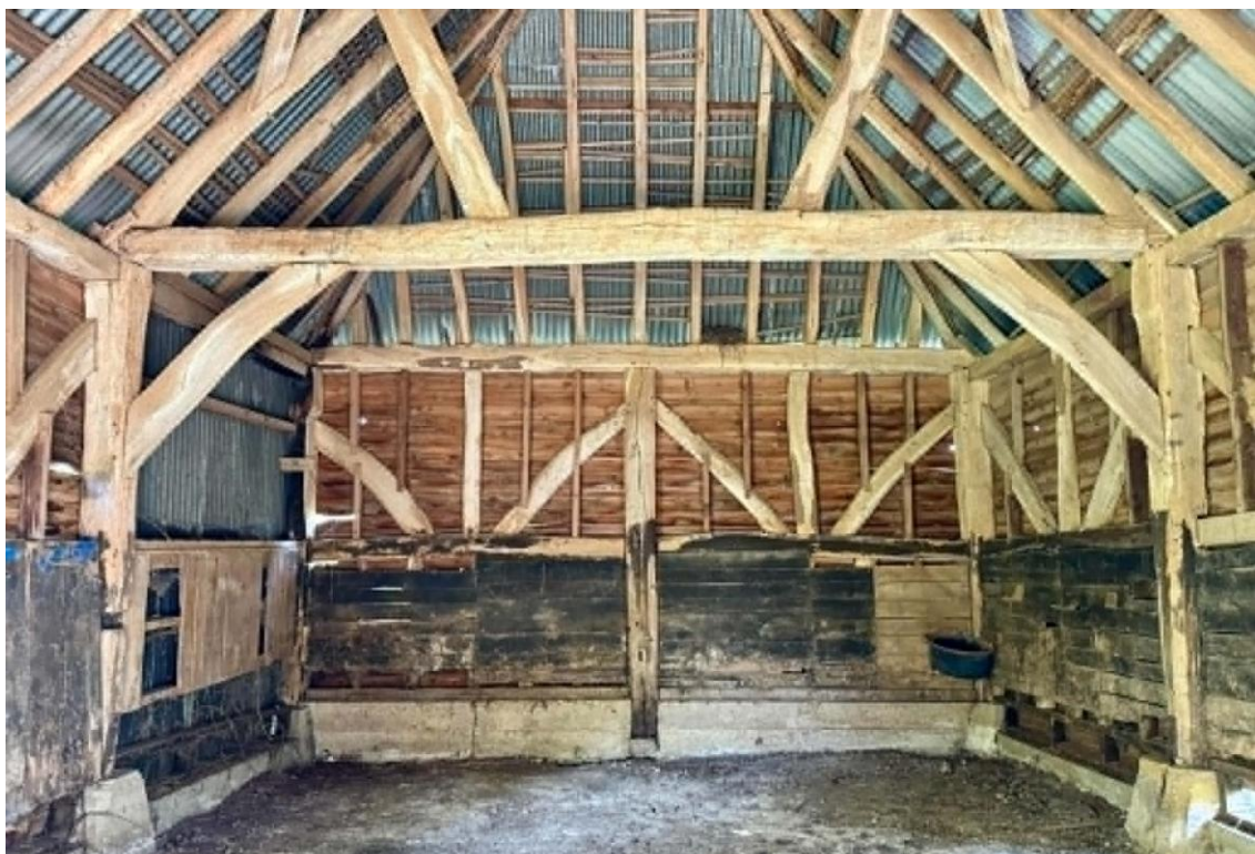
Fig 6: The tithe barn has a modern concrete dwarf wall all round, having been assembled on site in the early 20 th Century. The main timber frame is largely 17 th Century with early 20 th Century rafters, timber weatherboarding and corrugated metal roof sheeting. Left, metal sheeting covers the bay wall to the south-west corner that originally was built as an L-shape in that corner. New windows will be insert here.
