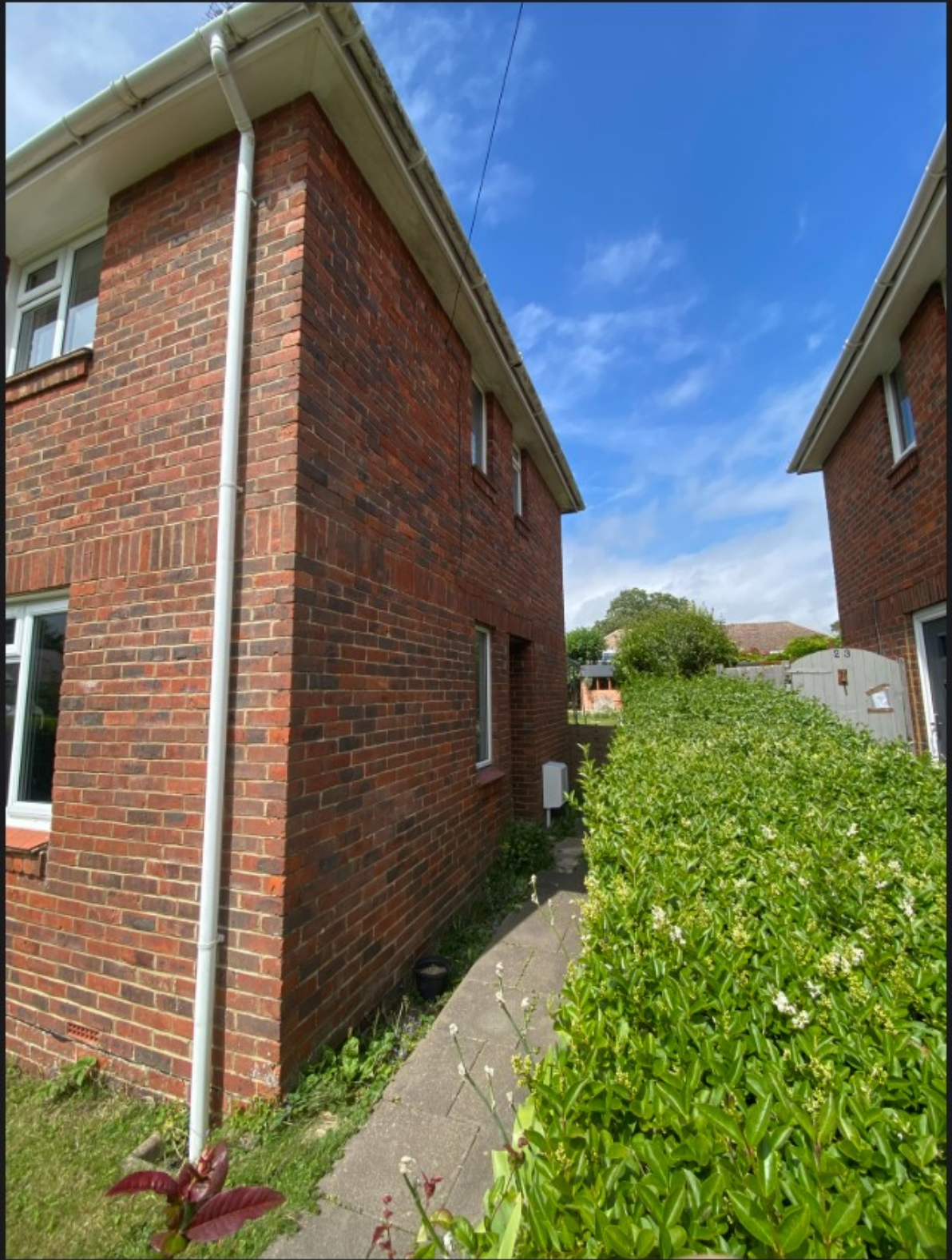
22 Priory Field Side Elevation - View 1
