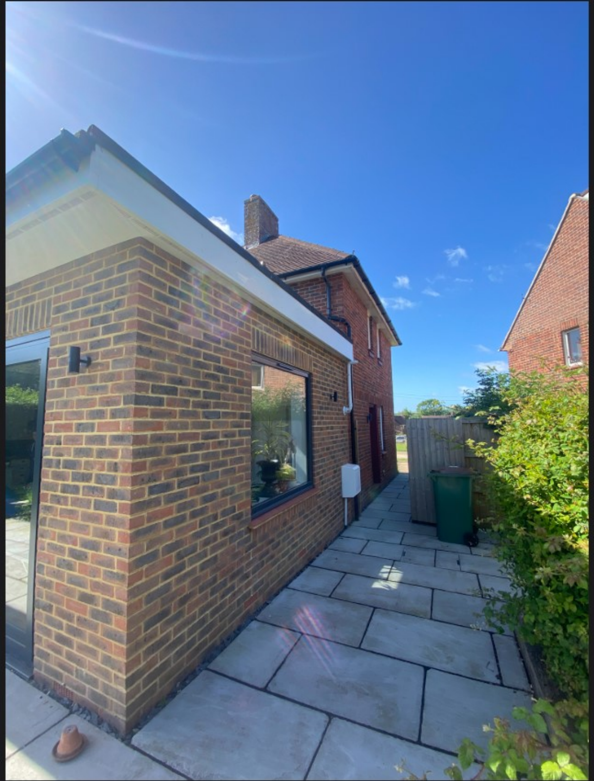
21 Priory Field Side Elevation – View 4
