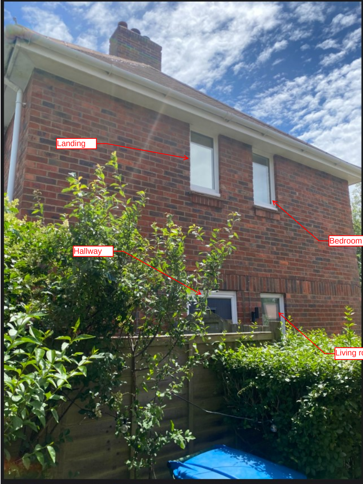
23 Priory Field Side Elevation – View 1
