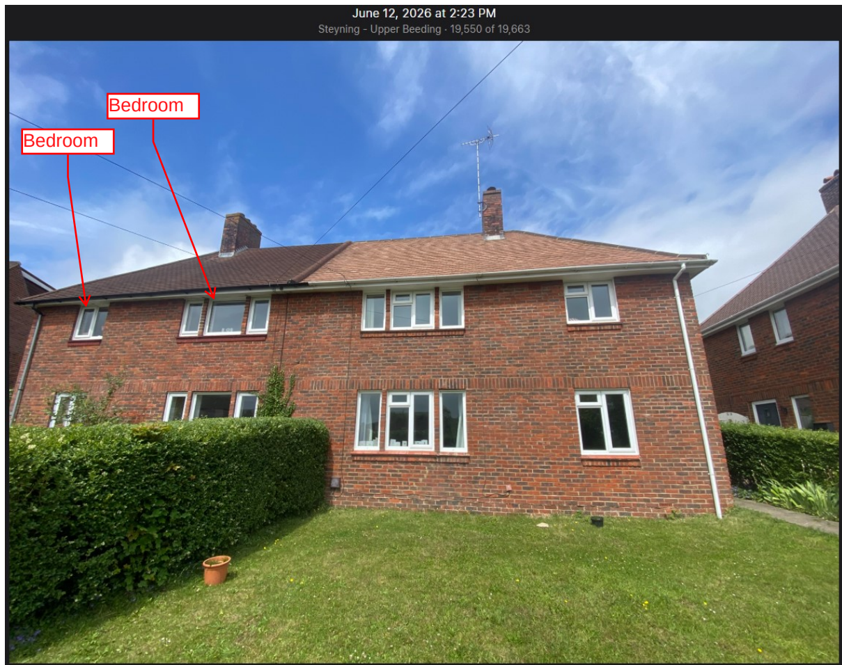
22 Priory Field Front Elevation and front garden, with front elevation of 21 Priory Field and side elevation of 23 Priory Field
