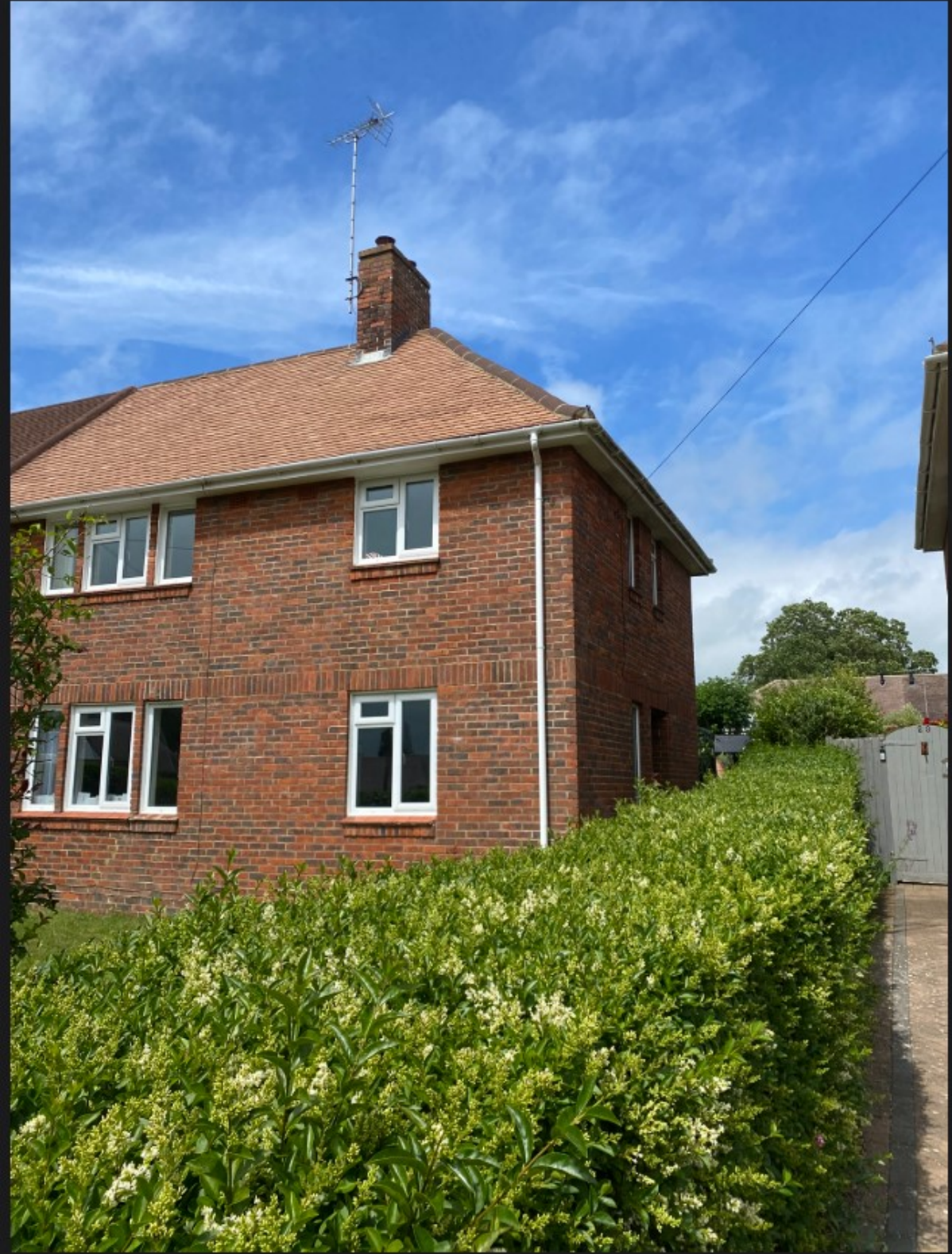
22 Priory Field Side Elevation - View 2
