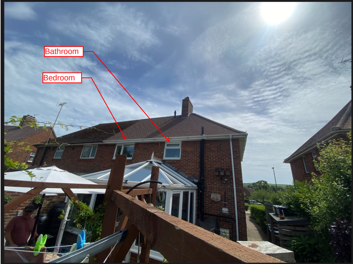
23 Priory Field Rear Elevation – View 2
