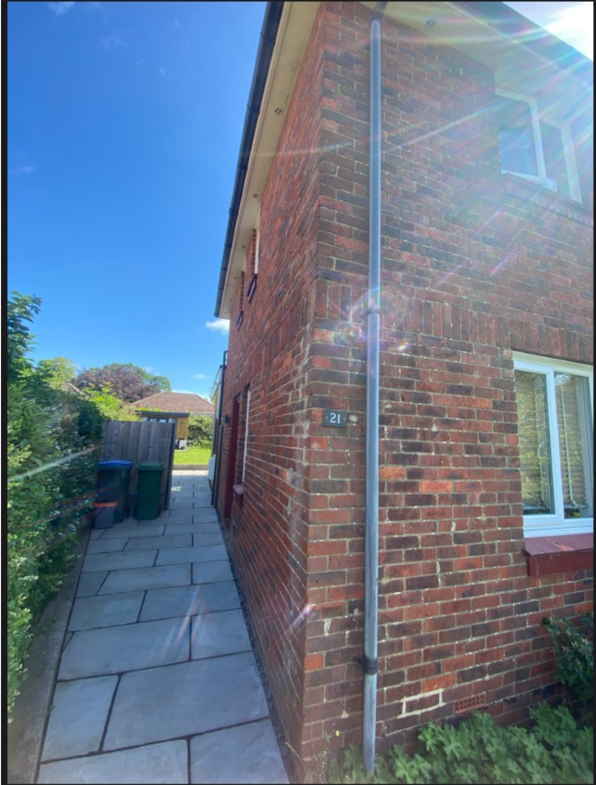
21 Priory Field Side Elevation – View 1
