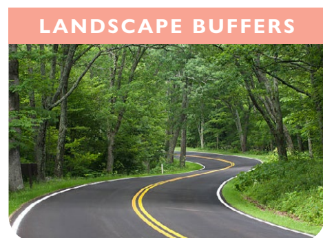
Woodland edge along primary road
