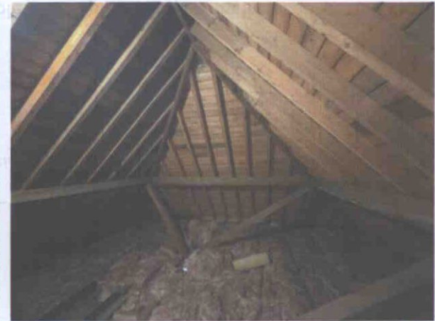
Building B1 - internal void
