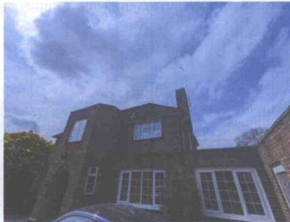
Building B1 - northeast aspect
