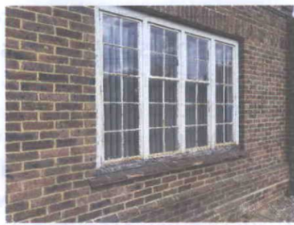
Examples of poor condition of the single glazing
