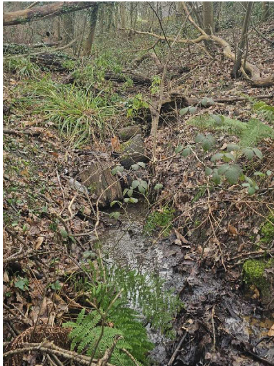
Image 28: Looking south, back up the ditch Logs blocking ditch before it intersects the ditch running West / East Adjacent the A283
