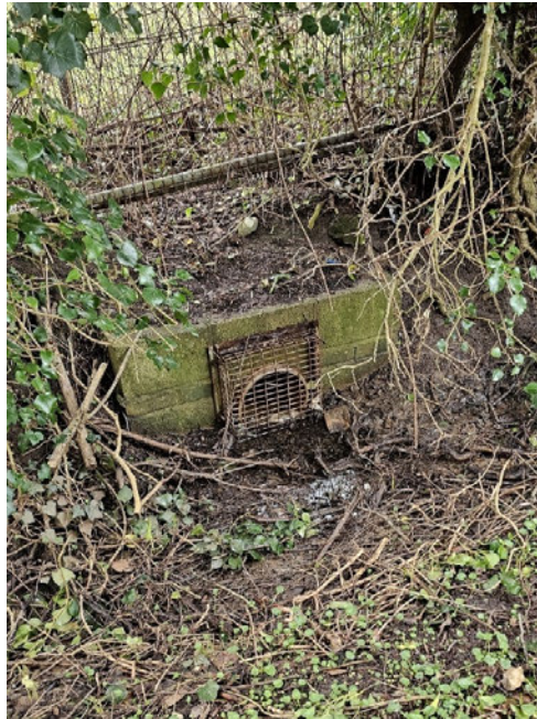
Image 02: 300mm diameter surface water outfall
