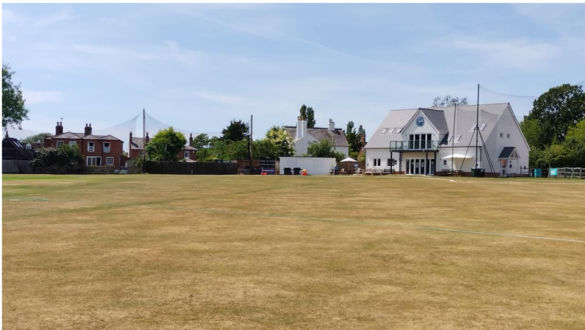
Figure 6: View of the new storage shed, from the cricket field. Forge Cottage (not listed) is visible on the left side of the photograph, the pavilion on the right side. Forge House can just be seen behind the tree and wall, between the shed and Forge Cottage.
