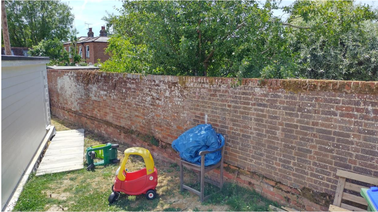
Figure 3: The wall behind the storage shed, which marks the boundary of the Conservation Area
