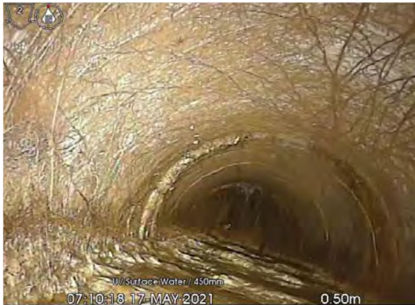
S 21X_8c00149b-c37e-4b90-9d39-705429272385_20210518_1 55156_682.jpg, 00:00:34, 0.50 m Settled deposits, hard or compacted, 40% cross-sectional area loss
