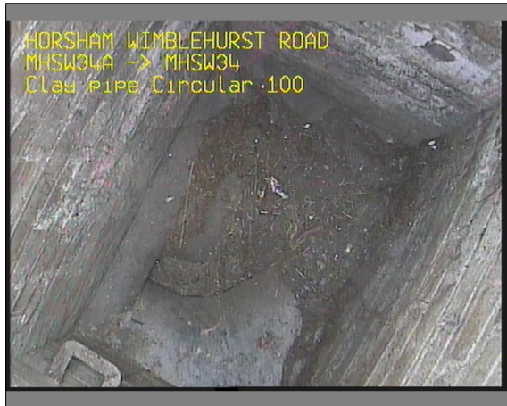
Photo: 36_36_226_A.JPG 0.02m, Start node type, manhole, reference number : MHSW34A
