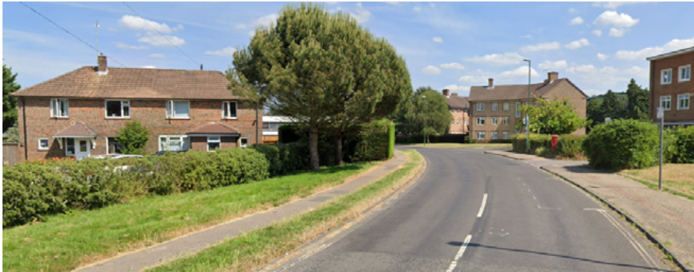
1. APPROACH FROM NORTH SIDE OF BLACKBRIDGE LANE
