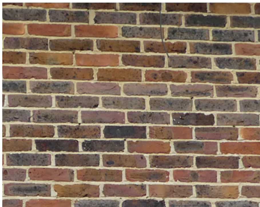
1 WALLS IBSTOCK CHAILEY RUSTIC BRICKS TO MATCH BRICKS ON EXISTING HOUSE
