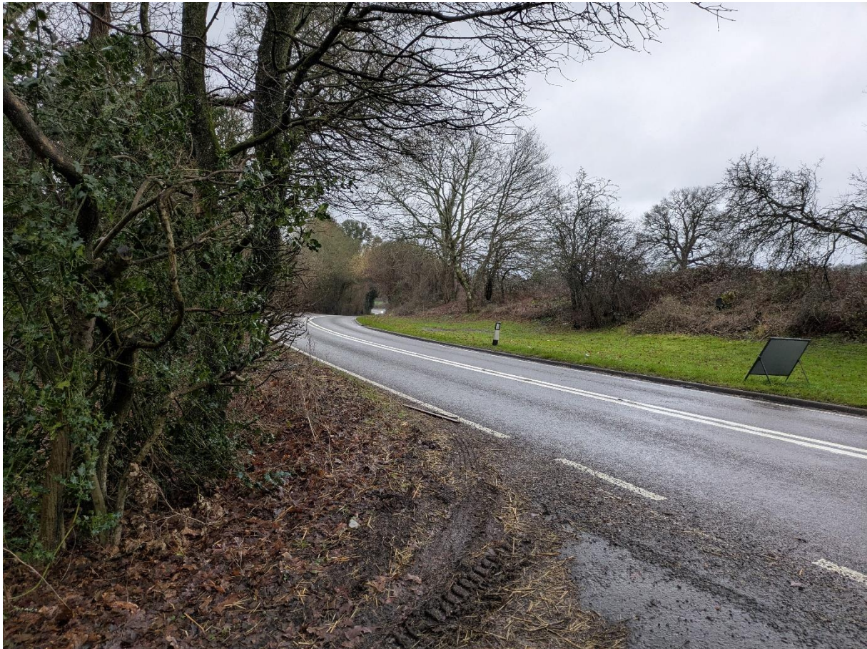
Figure 2 - View looking left from the access
