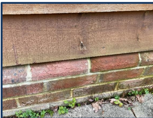
Photo 7 – Brick and mortar
