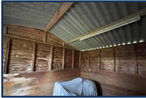
Photo 15 – Stable block interior
