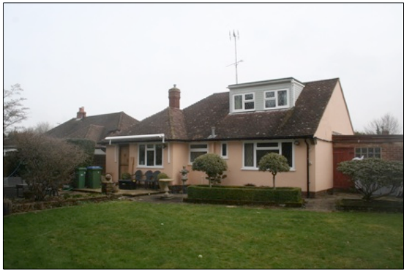
Rear elevation of number 22
