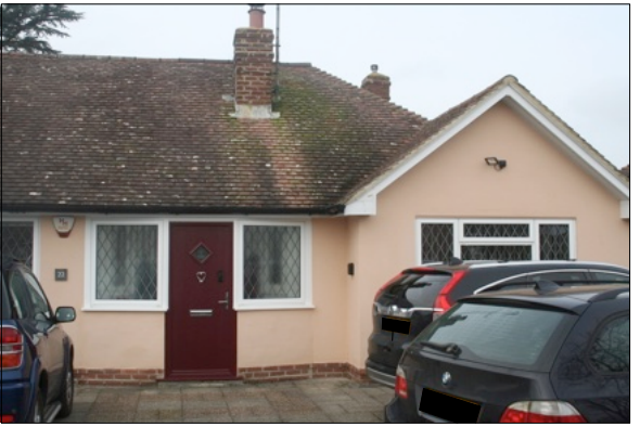
Front elevation of number 22
