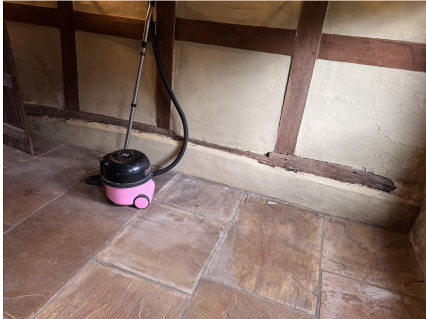
Photo (viii) – timber ground beam to dining room encased in mortar
