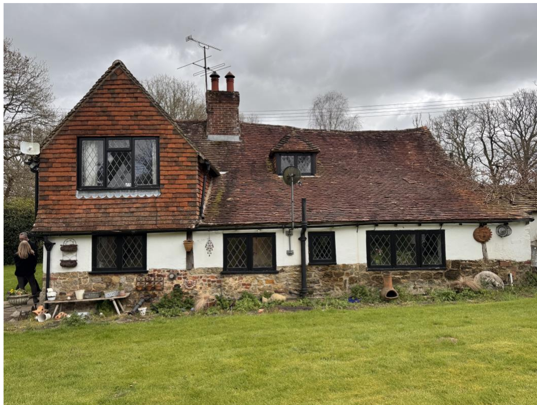
Photo (ii) – rear elevation
