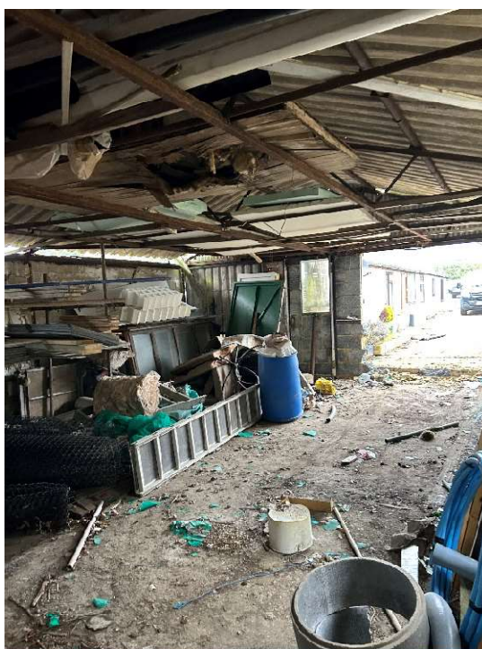
Photo 4: Northern room of the western warehouse section.
