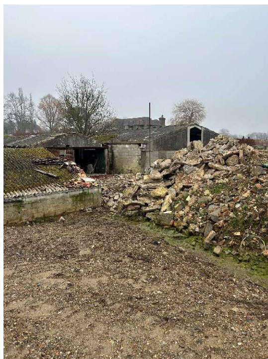
Photo 1: View of workshop building from former yard to the south, with reprofied soil and piled hardcore.
