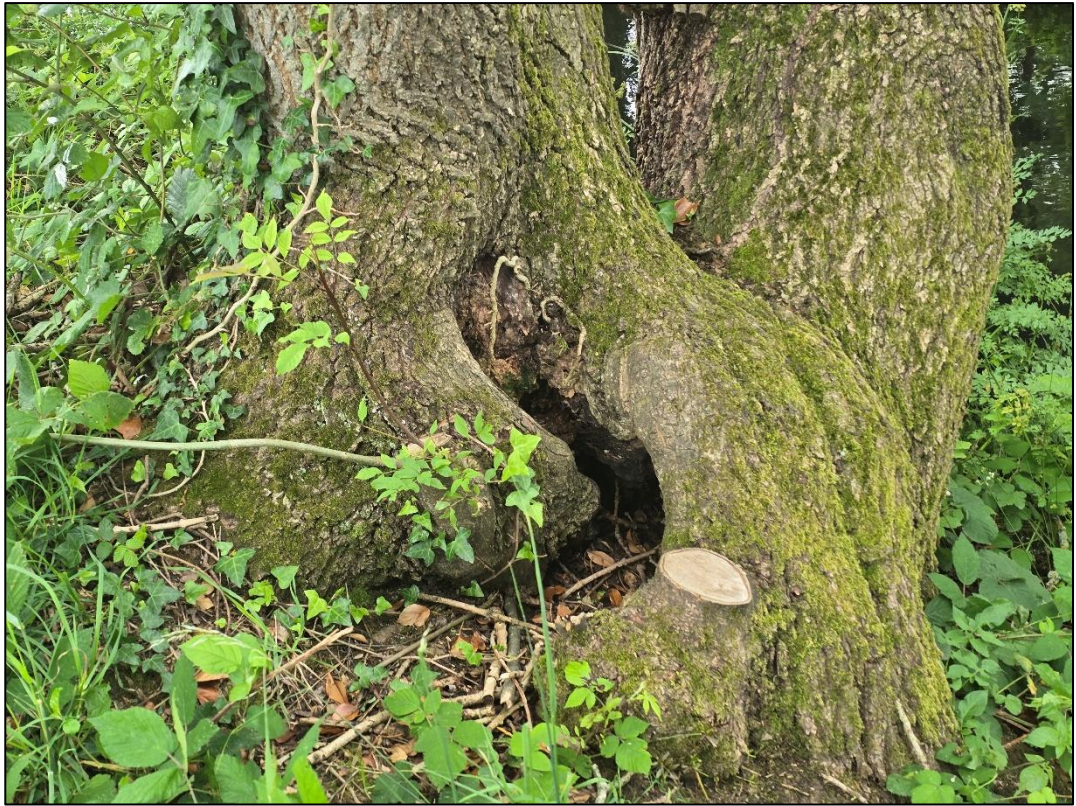
Photo 3 – Cavity / decay at the base of T253 (Ash)
