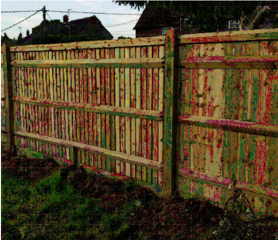
TIMBER CLOSE BOARD FENCE
