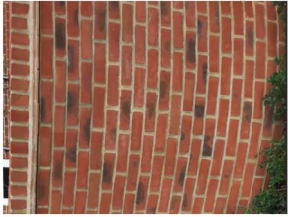
SCREEN WALL (Brickwork)
