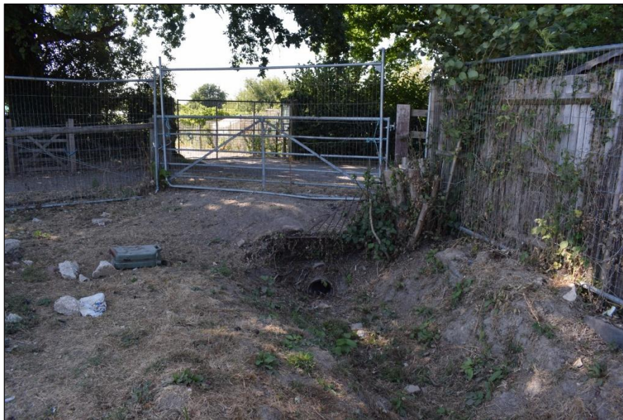
Plate 8. Drainage ditch and outflow in north-west corner of site
