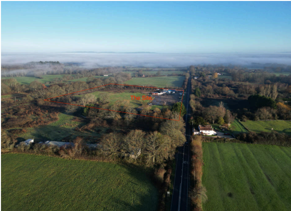
Aerial shot looking north across the site.
