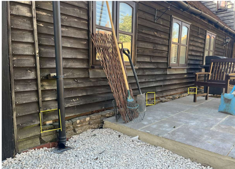
Figure 1 – The steel columns are visible above plinth level.
