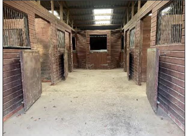
Plate 8: Internal of the barn.
