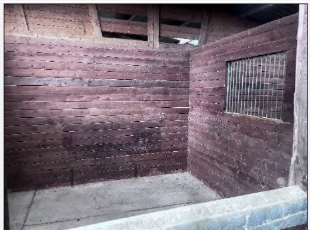
Plate 6: Internal of the barn.
