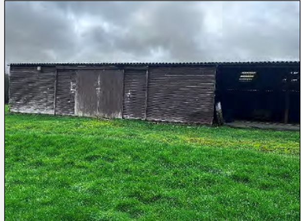
Plate 2: Northwest elevation of the barn.
