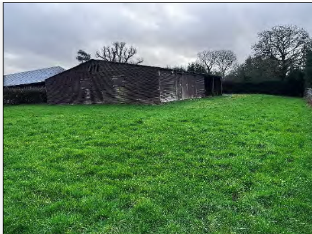
Plate 3: Facing south from the north corner.
