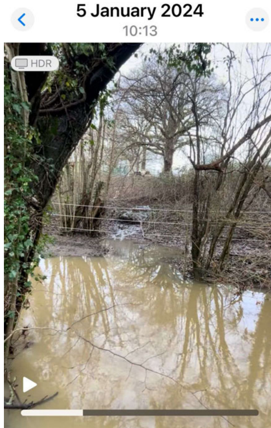
Still from a Video of the Same Manhole from the Other Bank of Parsons Brook
