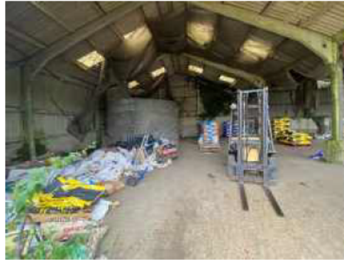
Tank within structure
