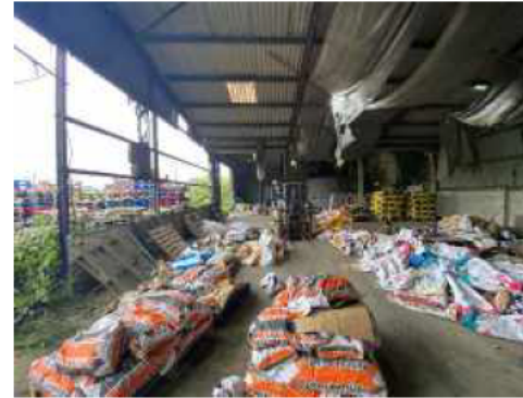
Bags of potatoes stored within the structure
