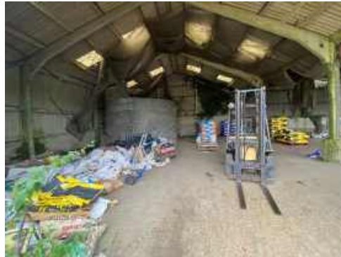
Tank within structure
