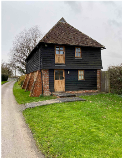
Existing North elevation of the Granary:
