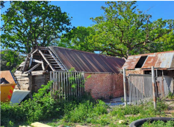
Photo 3: Displaying gaps between ridge beams.
