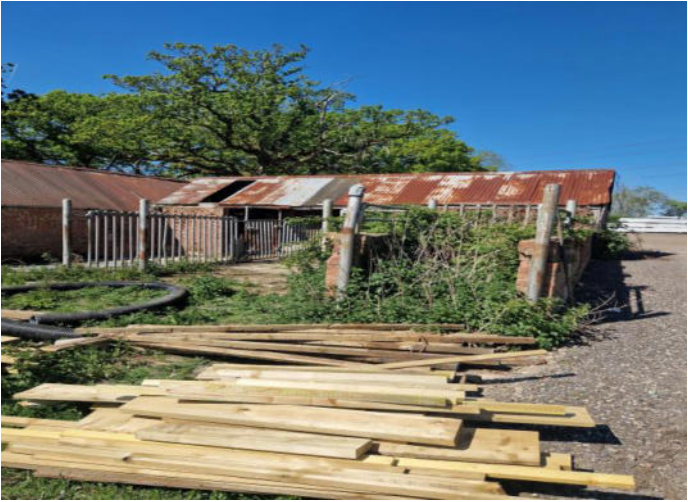
Photo 6: Displaying gaps in roofing sheets and open southern aspect.
