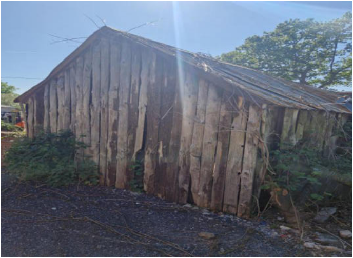
Photo 6: Displaying gaps in roofing sheets and open southern aspect.
