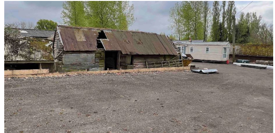
Figure 2.2 - Existing Site Photographs
