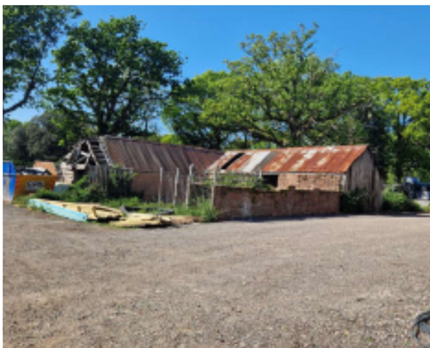
Figure 11: View of the site from the south-east corner
