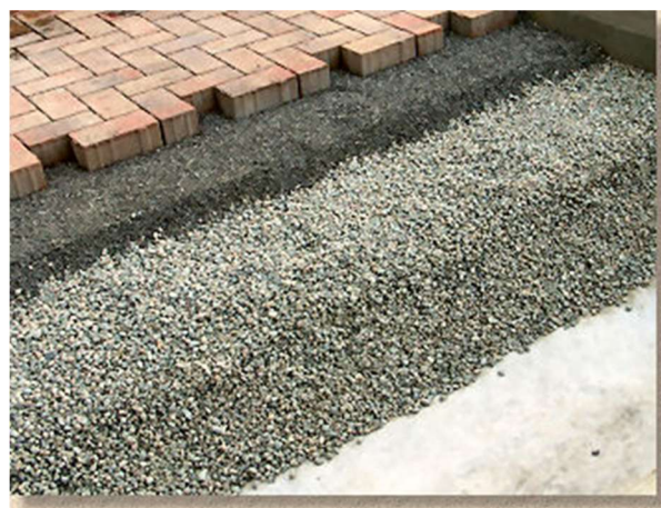
Figure 10: Typical permeable paving solution
