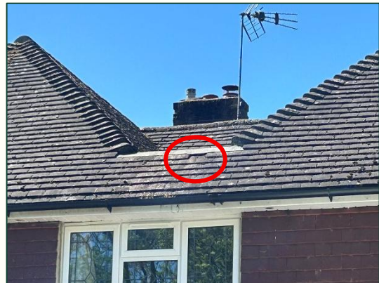
B1: Missing tile on the northern elevation
