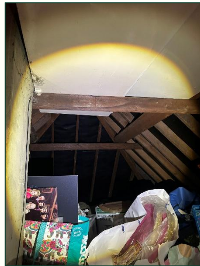
B1: Southern internal loft void
