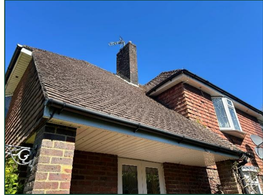
B1: Missing tile on the northern elevation
