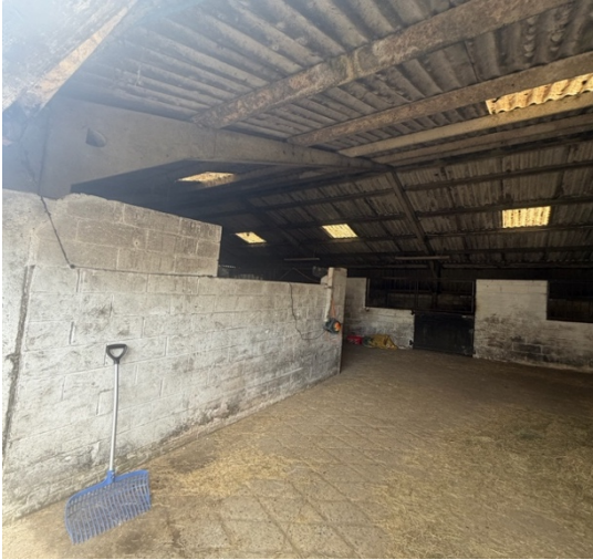
Plate 7: Internal View of Stables
