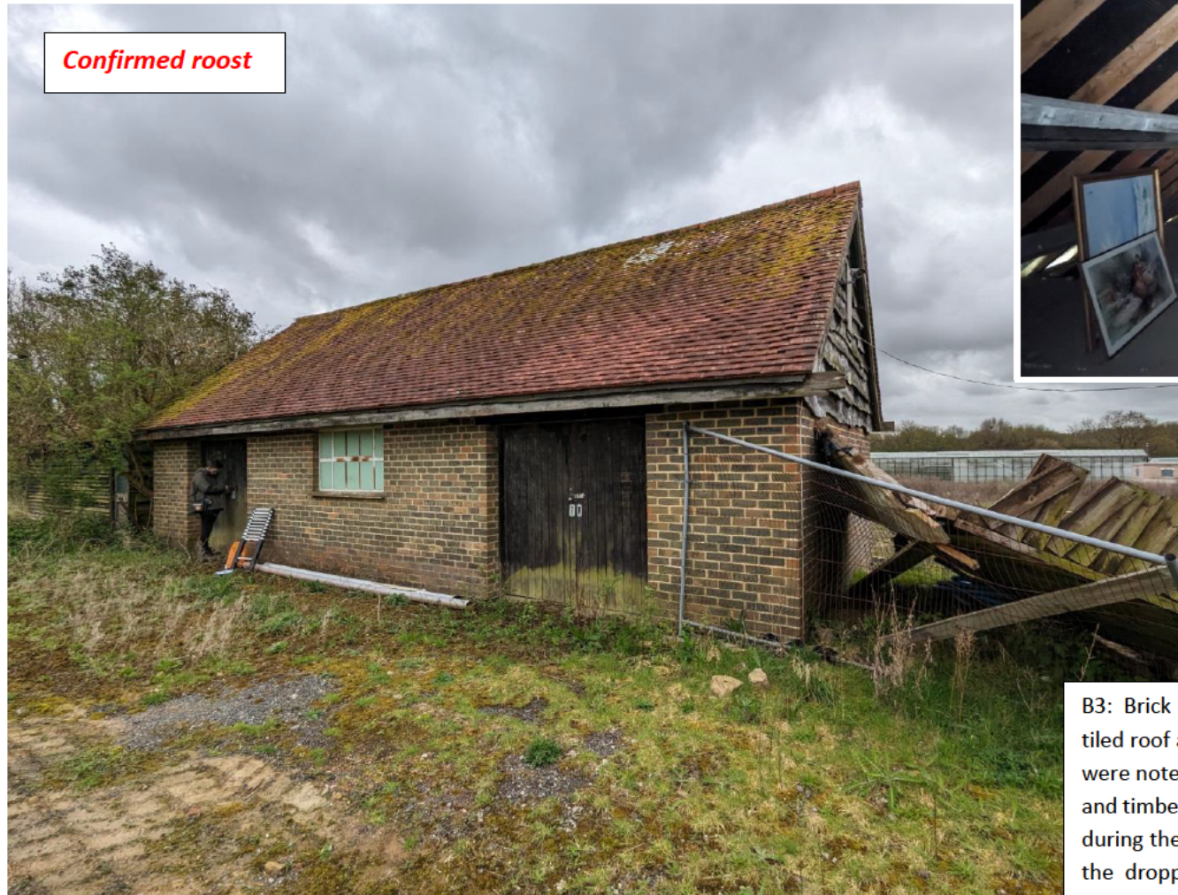
Figure 7. Preliminary roost assessment of Building 3 on site (taken April 2024).
