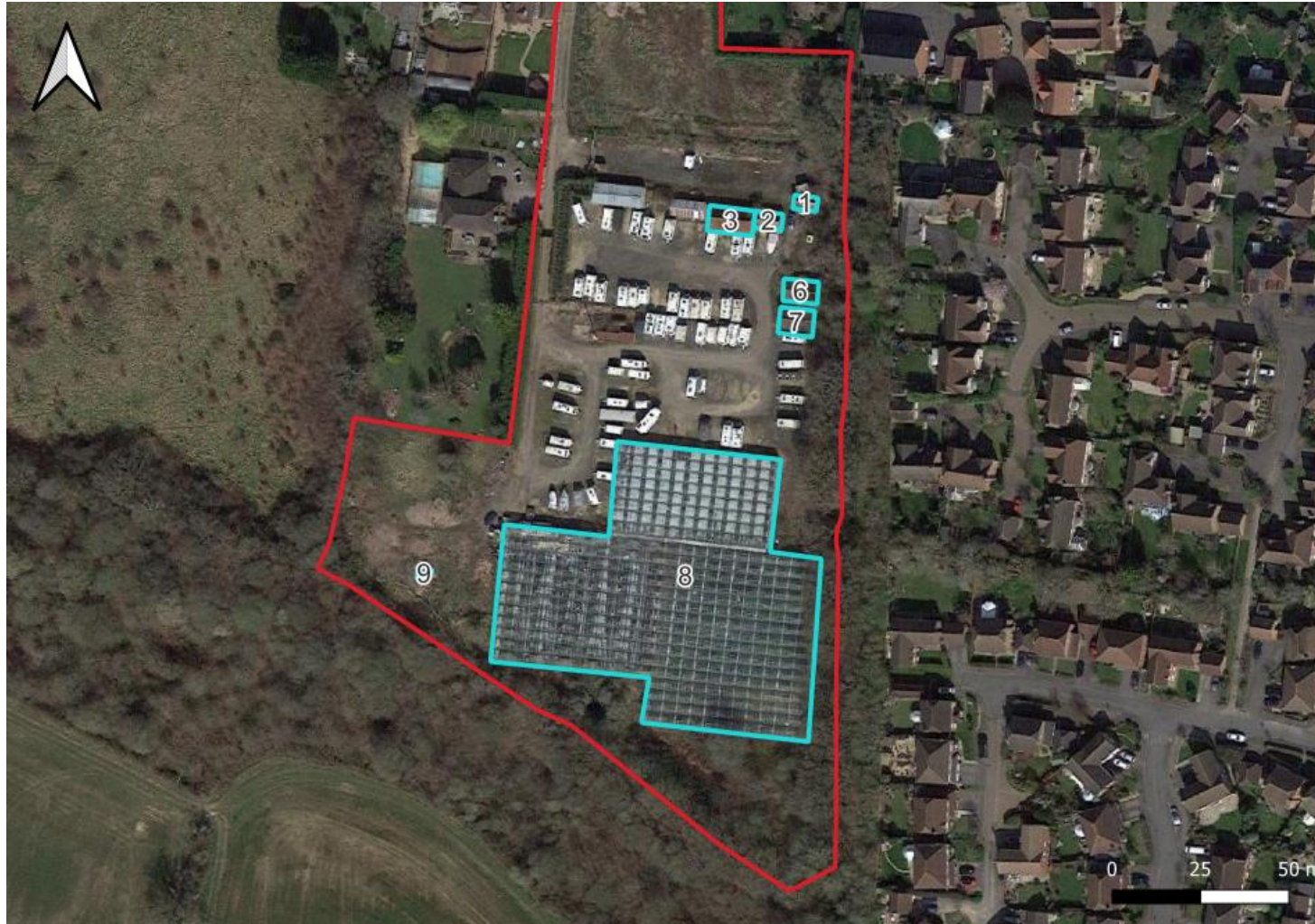
Figure 6. Location of the 7 buildings still present on site (Buildings 4 and 5 are not indicated as these had become completely dilapidated and collapsed) (Google Satellite, 2024).
