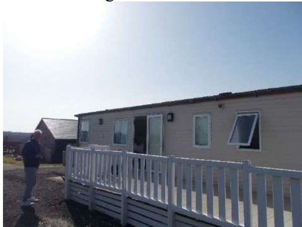
Existing caravan to the east
