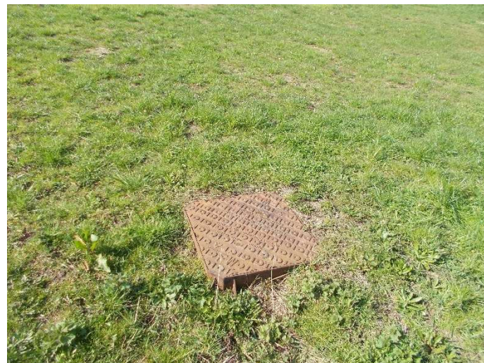
Existing manhole leading from sewage treatment plant
