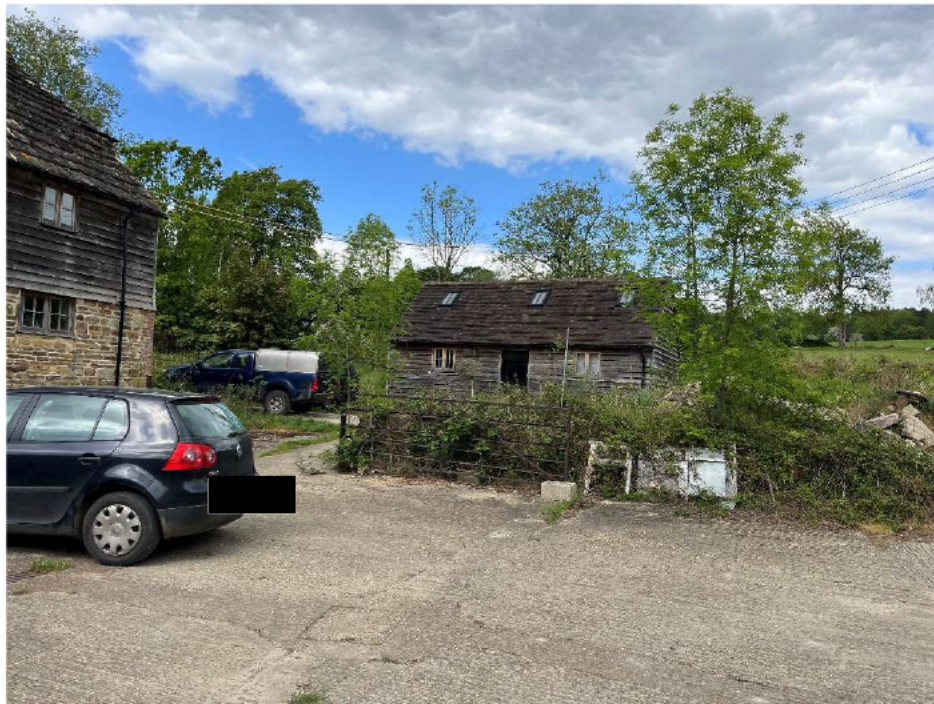
Views of the application building and access from the original farmyard.
