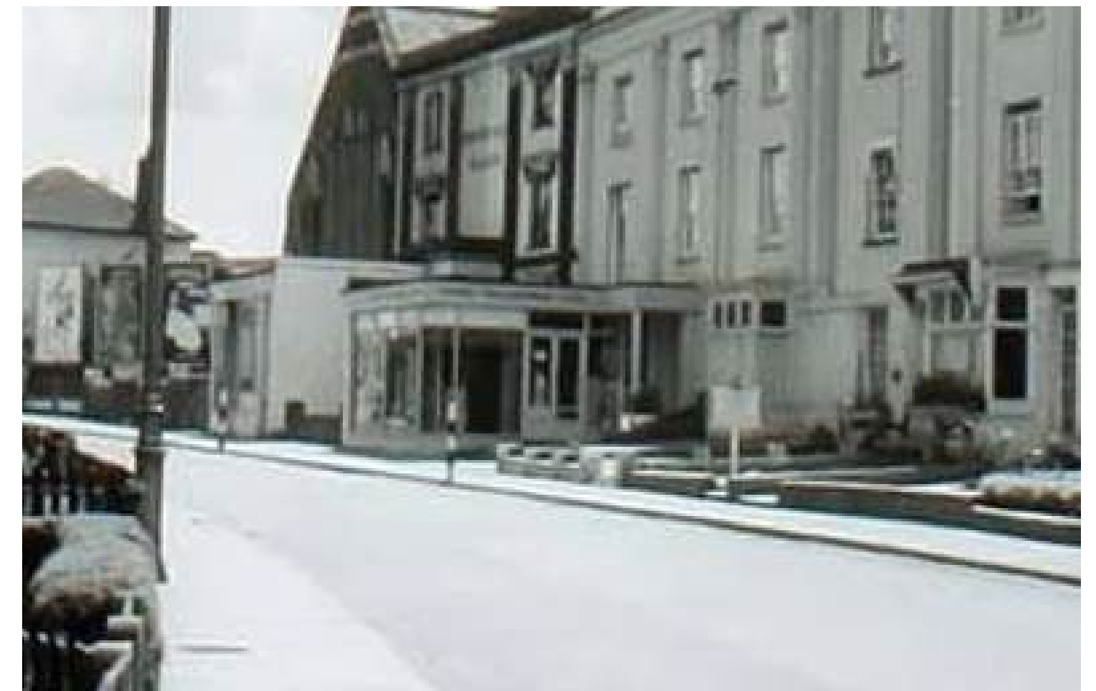
Figure 10 - Extract from 1960 record photographs showing No.47 with shopfront, from the north, centre of picture. (Historic England, 2026)
