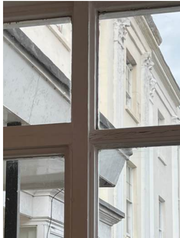
New partition to abut original shopfront mullion.
