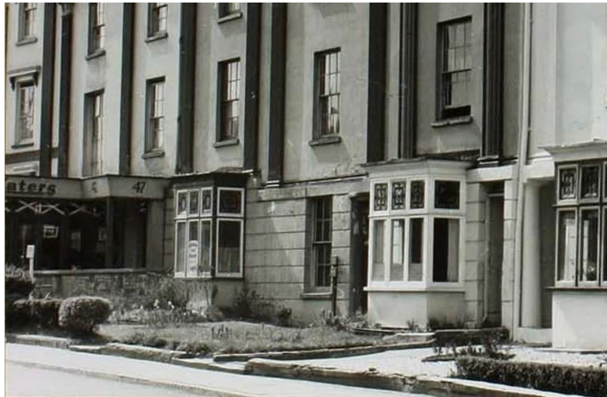
Figure 7 - Extract from 1950 record photographs showing No.47 with shopfront, from the southeast, centre of picture. (Historic England, 2026)
