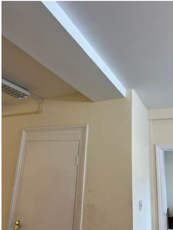
New partition to sit under ceiling beam on line of original house frontage.
