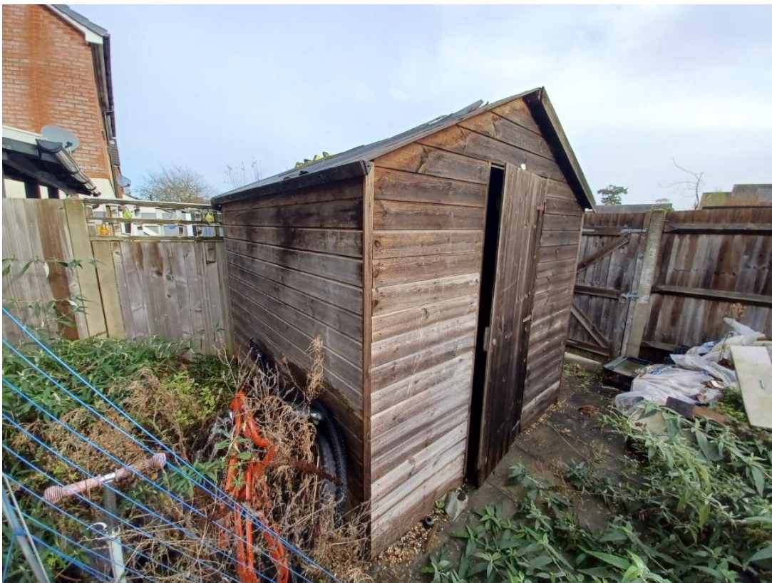
Figure 1: Original shed taken from neighbouring property at Reeves Court
