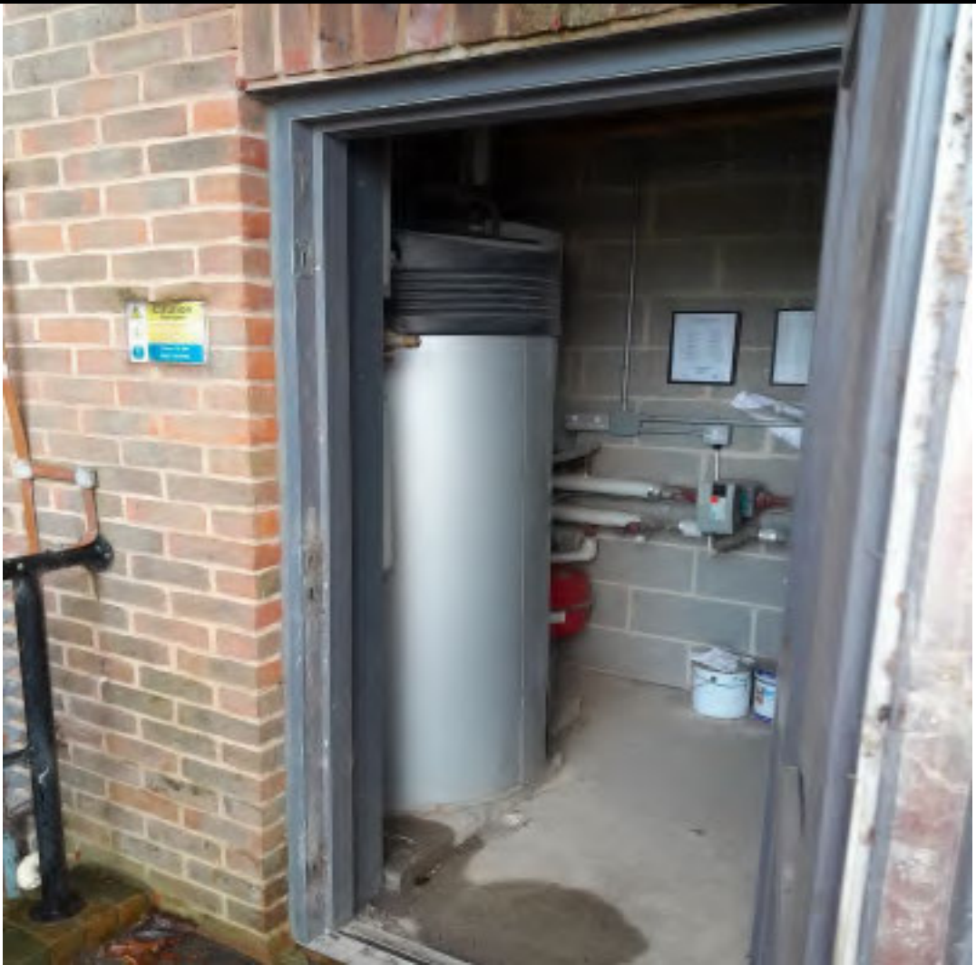
Plate 5 –Boiler Room associated with pavilion (EFAG)PI on the Western border of Site – Looking West
