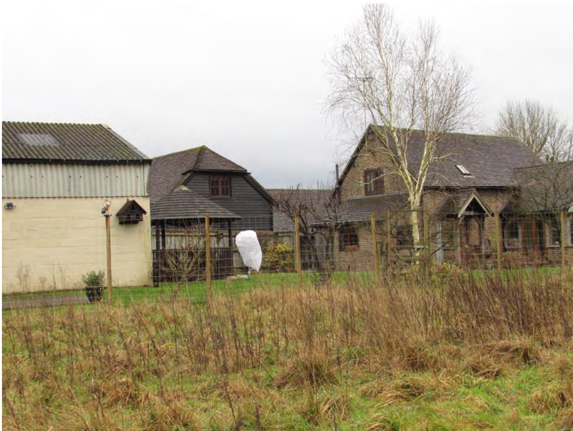
Plate 4: View of the Southern Two Buildings at Hornbrook Farm Looking Southeast
