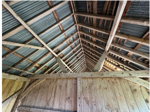
Photograph 2. Interior of the new section of the barn.
