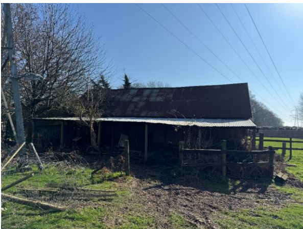
Photograph 5. The lean-to section of the barn.
