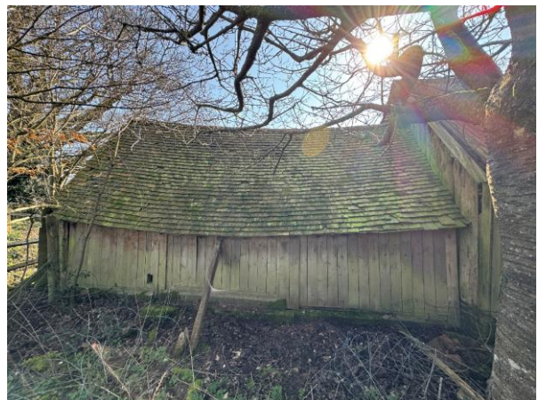
Photograph 6. The barn viewed from the north.
