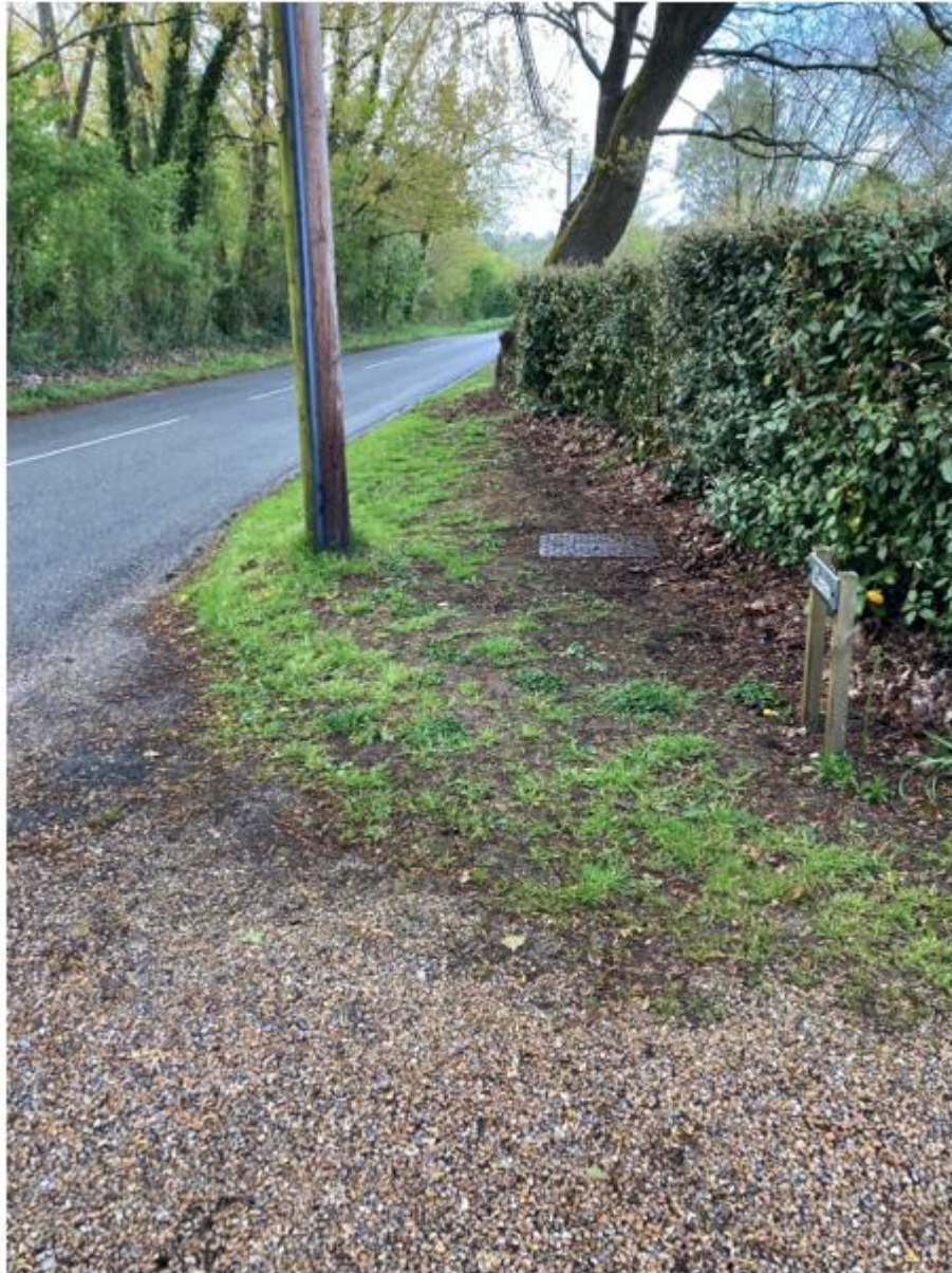
Figure 1 – Existing access north splay at 2.4 metres
