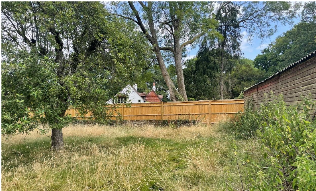
Figure 12: Views to the listed building from the rear of the application site where the listed building can be seen beyond the existing boundary treatment.
