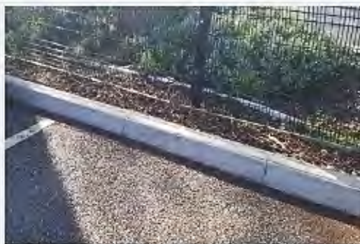
Standard kerbs set on top of concrete-filled geocells
