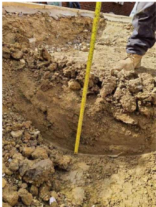
Pit excavated into formation level of Plot 7
