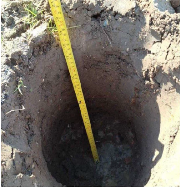
Inspection pit POSHP2 in Central Area on 30 th September 2025 showing 200mm topsoil and 250mm subsoil with formation level soils at the base
