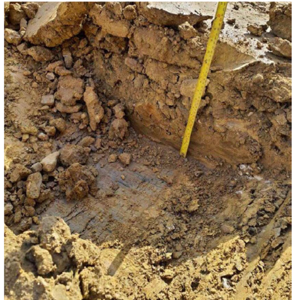
Inspection pit excavated 350mm into the formation level
