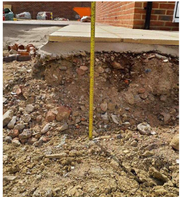
Tape measure showing reduction in formation level 400mm below final level (from patio) in Plot 13
