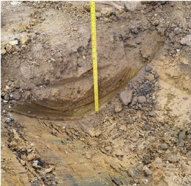
Inspection pit excavated 450mm into the formation level, indicating made ground was present in the formation level soils
