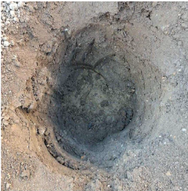
Inspection Pit in Plot 12 showing Formation Level soils at the base of the pit
