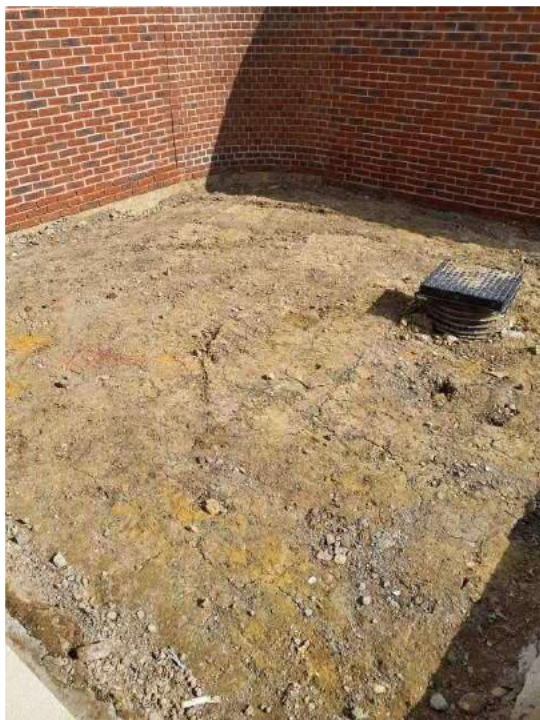
View of formation level of Plot 7
