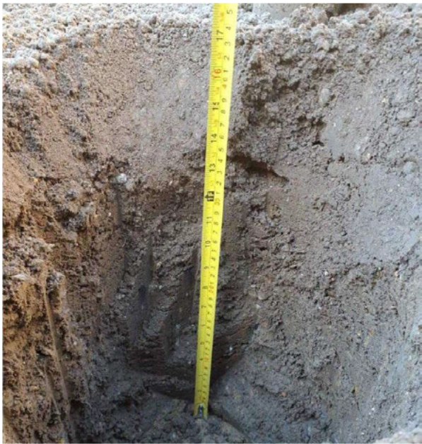
Inspection Pit in Plot 12 showing 400mm of Topsoil and Formation Soils at the Base
