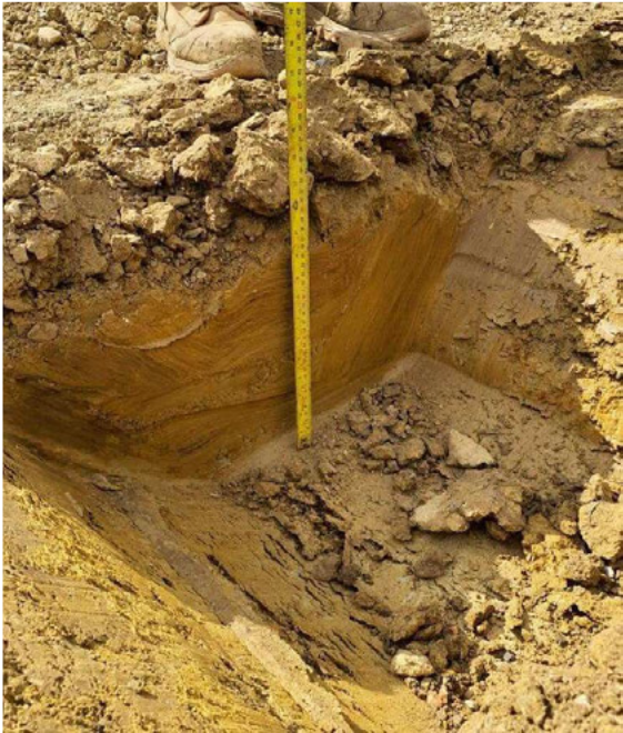
Inspection pit excavated 400mm into formation level of Plot 13
