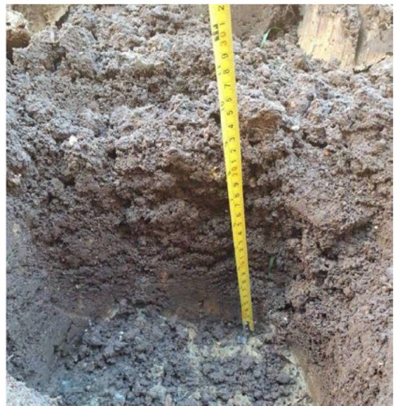
Inspection Pit in Plot 5 showing 300mm of Topsoil and Formation Soils Beneath
