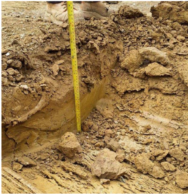
Inspection pit excavated 400mm in Plot 12
