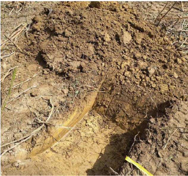
Inspection pit in formation level in Plot 8
