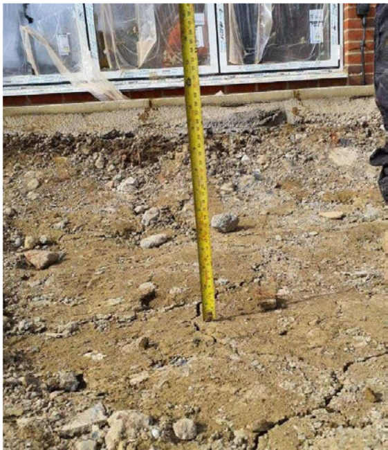
Tape measure showing reduction in formation level by 300mm
