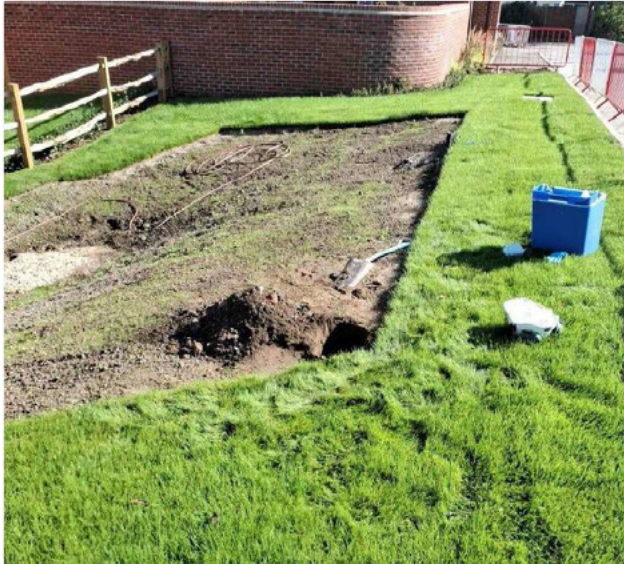
Central Area on 30 th September 2025 showing topsoil and turf placed
