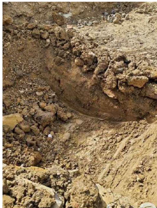
Pit excavated into formation level of Plot 7
